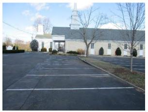
Rain gardens can be installed to capture, treat, and infiltrate stormwater runoff from sections of the roof. A section of parking spaces can be converted to porous pavement to capture and infiltrate runoff from the parking lot. A cistern can be installed to capture rooftop runoff and provide water for watering gardens or other non-potable uses. A preliminary soil assessment suggests that more soil testing would be required before determining the soil's suitability for green infrastructure.
