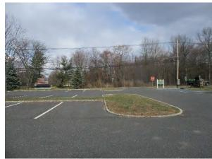
Two sections of parking spaces can be converted to porous pavement to capture and infiltrate stormwater runoff from the parking lot. A preliminary soil assessment suggests that more soil testing would be required before determining the soil's suitability for green infrastructure.
