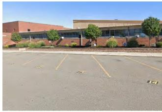
The existing parking spaces to the south of the school can be converted into pervious pavement to capture and infiltrate the stormwater runoff from the asphalt. Trench drains will be required. The downspouts on the southern side of the building can also be disconnected to the pervious pavement to manage rooftop runoff. A preliminary soil assessment suggests that more soil testing would be required before determining the soil's suitability for green infrastructure.
