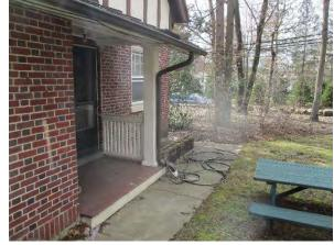
Rain gardens can be installed in the turfgrass area near the entrance of the building and in the rear to capture, treat, and infiltrate stormwater runoff from the parking lot. Downspout planter boxes can be installed to capture and treat stormwater runoff form the rooftop. A preliminary soil assessment suggests that more soil testing would be required before determining the soil's suitability for green infrastructure.
