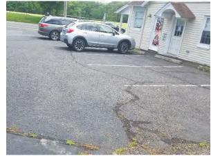
Parking spaces in the parking lot to the north of the building can be converted to porous pavement to capture and infiltrate stormwater runoff from the parking lot and roof. The downspout on the front of the building can be directed to downspout planter boxes to help capture stormwater. A preliminary soil assessment suggests that the soils have suitable drainage characteristics for green infrastructure.
