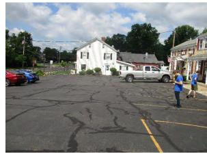
Parking spaces located in the south section of the parking lot can be replaced with pervious pavement to capture and infiltrate stormwater. Downspouts at Annie's Deli can be disconnected and directed into downspout planter boxes to capture and filter rooftop runoff. A preliminary soil assessment suggests that more soil testing would be required before determining the soil's suitability for green infrastructure.
