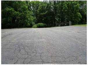
Pervious pavement can be installed in the northeast portion of the parking lot to capture and infiltrate stormwater runoff from the parking area. A preliminary soil assessment suggests that the soils have suitable drainage characteristics for green infrastructure.
