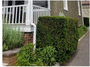
Downspouts on the northwest and southeast corners of the building can be disconnected and converted to planter boxes to capture stormwater runoff from the roof. A preliminary soil assessment suggests that more soil testing would be required before determining the soil's suitability for green infrastructure.
