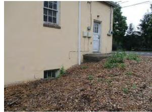
A rain garden can be installed on the east side of the building to capture, treat, and infiltrate rooftop runoff. Along the western side of the building a downspout planter box can be installed to help capture stormwater runoff. A preliminary soil assessment suggests that more soil testing would be required before determining the soil's suitability for green infrastructure.
