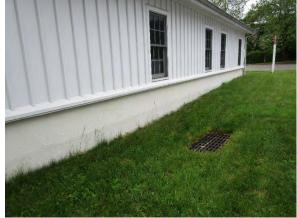
A rain garden can be installed near the rear entrance of the building to capture, treat, and infiltrate the water from five nearby connected downspouts. Two downspout planter boxes can be installed to capture rooftop runoff from different sections of the building. A preliminary soil assessment suggests that the soils have suitable drainage characteristics for green infrastructure.
