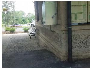
Downspouts on the north and south of the building can be disconnected and converted to planter boxes to capture stormwater runoff from the roof. Sections of parking spaces can be converted to porous pavement to capture and infiltrate stormwater runoff from the parking lot. A preliminary soil assessment suggests that more soil testing would be required before determining the soil's suitability for green infrastructure.
